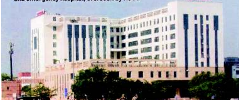
Safdarjung hospital, New Delhi, will get a super-specialty and emergency hospital, overseen by HSCC
