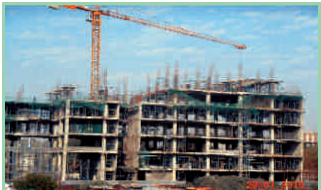
Construction of Super Speciality Block, Safdarjung Hospital, New Delhi
