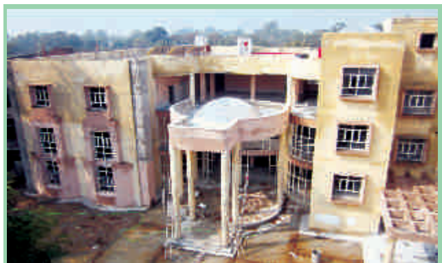
Construction of Nursing College at GMC, Patiala
