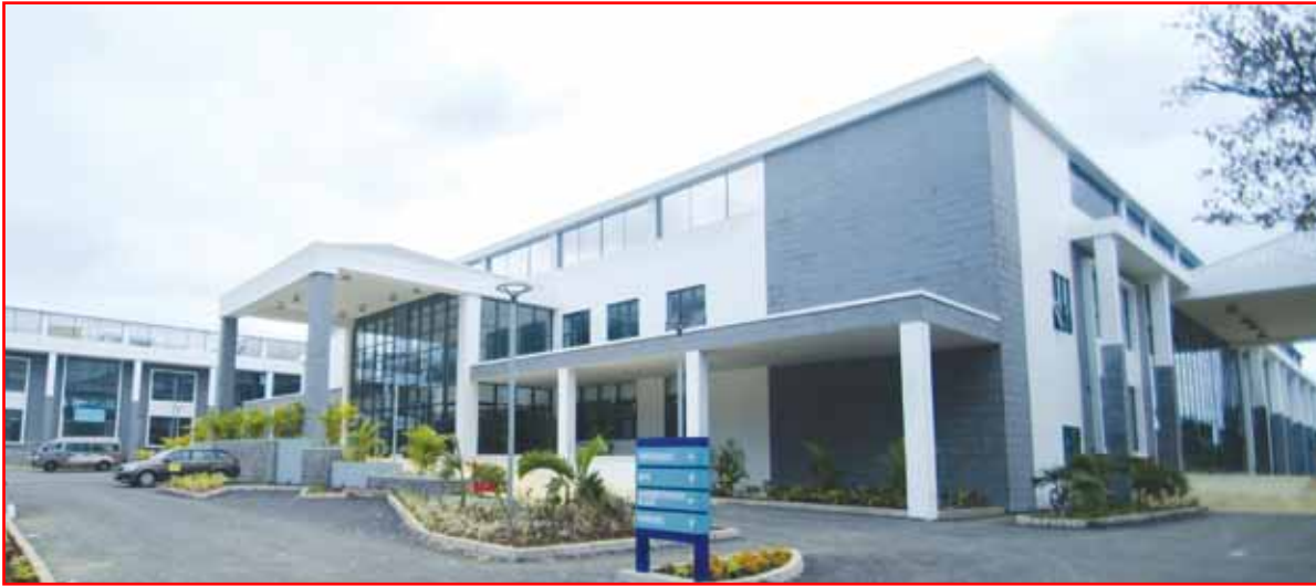
ENT Hospital at Mauritius
