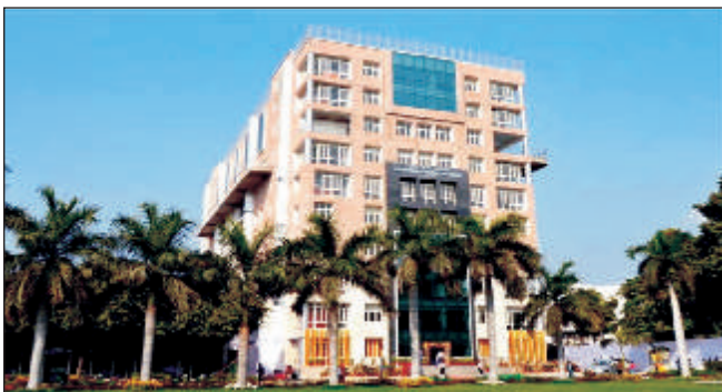
Convergence Centre, AIIMS
